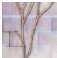
Termite mud tubes
